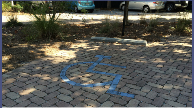
Permeable pavement in a parking lot
