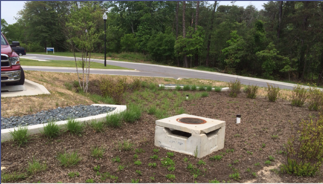
Bioretention with fore-bay
