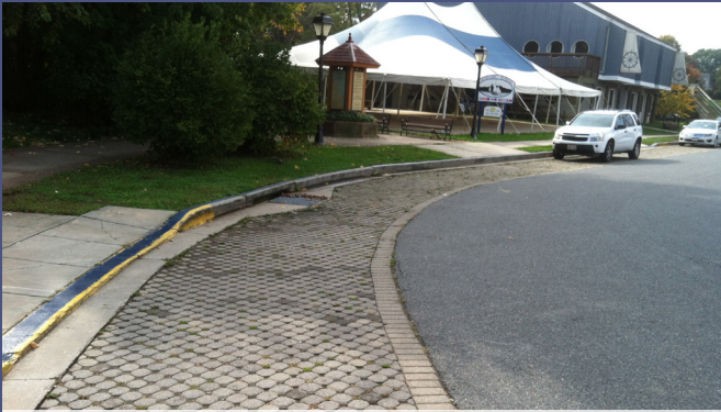
Permeable pavement for on-street parking
